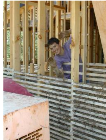
The cob walls
