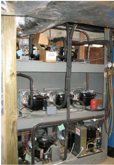
The water cooled compressors the heat recovery drain line
