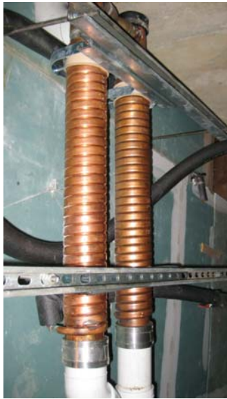
The water cooled compressors the heat recovery drain line
