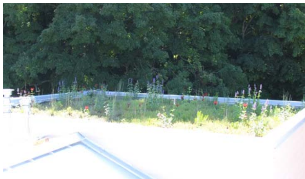
The green roof
